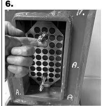
...and is placed flush with the back side of the transit. Hold the cover by hand...
