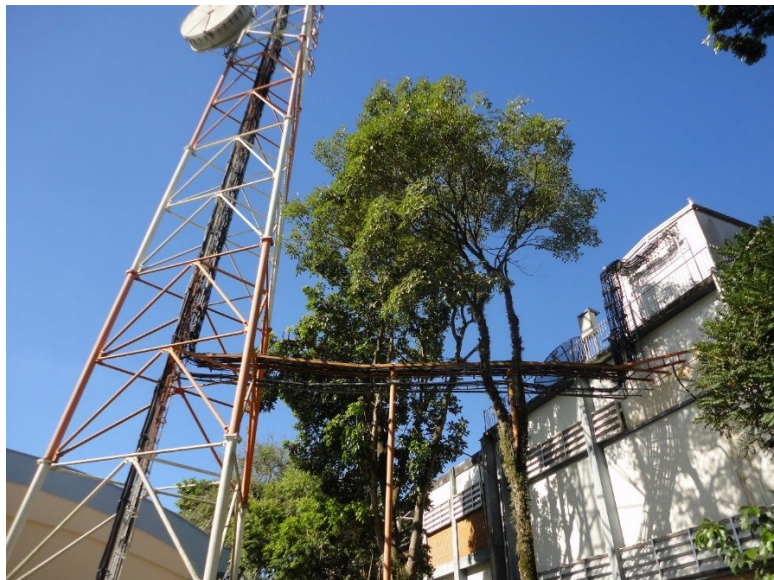
Figure 7a: Telecommunication installation where a large number of antenna cables can be seen entering the equipment room.
